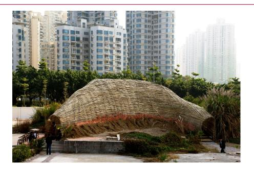
The building is realized on a wasteland of a ruined building site in between the Shenzen City Hall and an illegal workers camp. The design is inspired by insects. The bamboo construction methods are based on local knowledge from rural Guanxi brought into the city by migrating construction workers.
